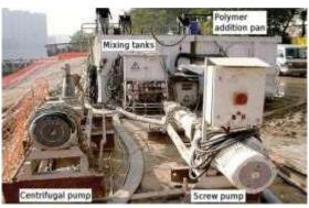
In the fluid circuit a screw pump and a centrifugal pump were used. The former was used to pump the polymer fluid from the tanks to the excavation, and the latter was used to return the used fluids to the tanks during concreting. The rationale for this arrangement is that polymer fluids are prone to damage by the high shear stresses induced by centrifugal pumps, hence the lower shear screw pump was used to
