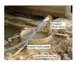
Prior to the excavation, a 10 m long temporary casing was inserted into the ground at each pile location to support the soft alluvial clay at the top. The pile bore was excavated dry to the bottom of the casing and then under the support of polymer fluid.
